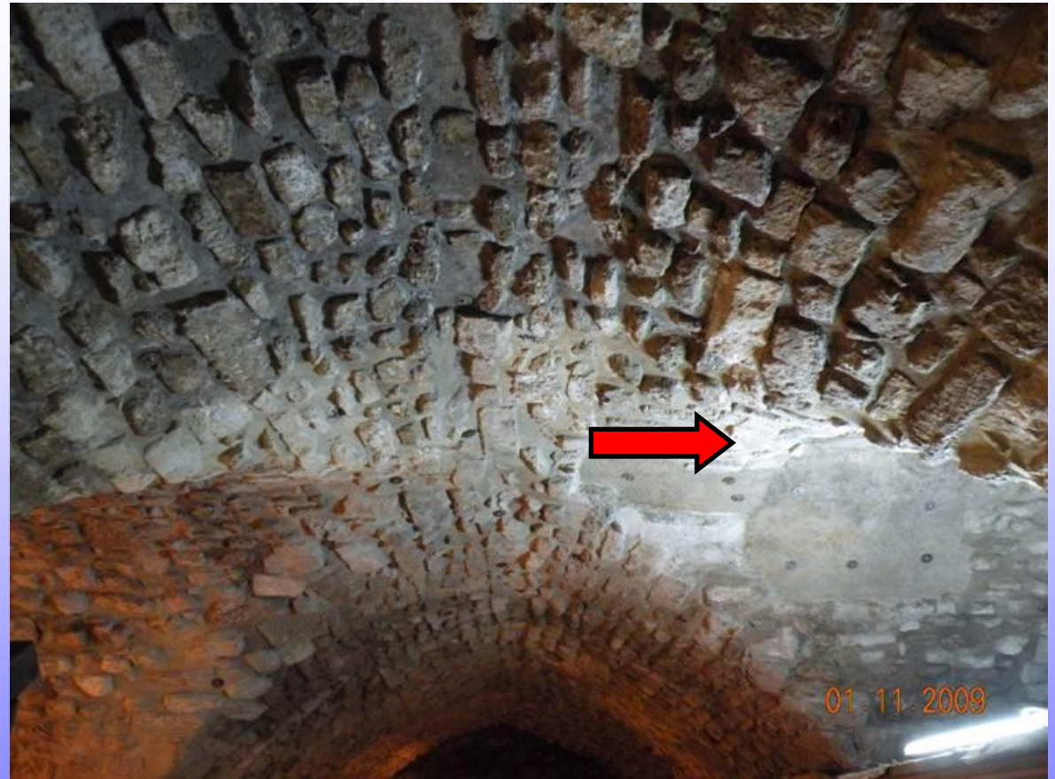
Lime based concrete casting
